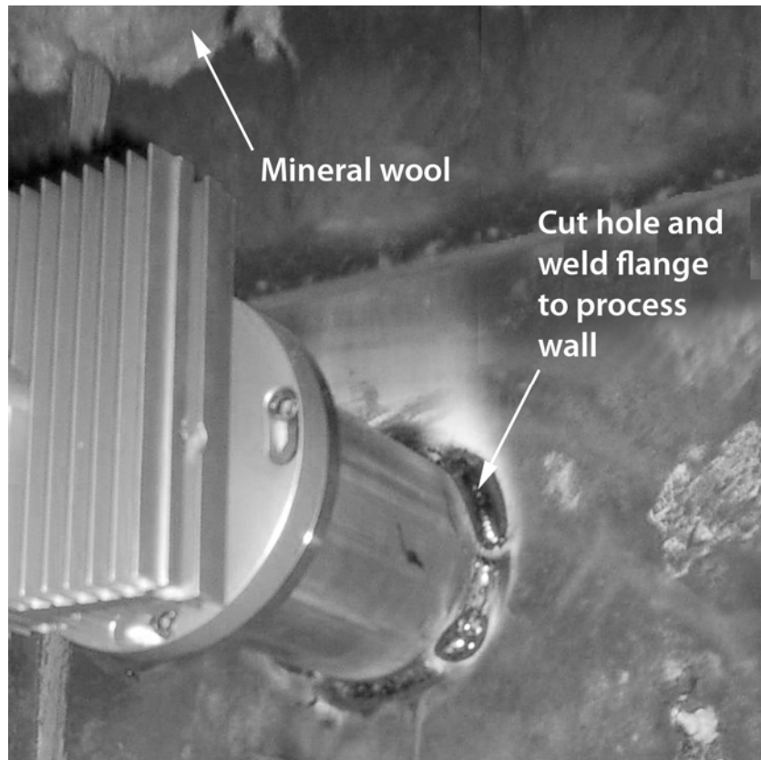
Figure 63 Cooling Set Installation
